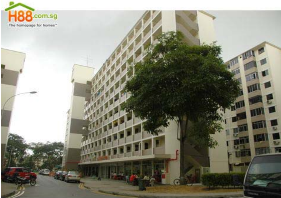
State of the flats before demolition
